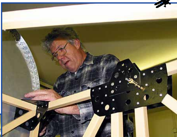
Ernie soloing on the firewall work.
