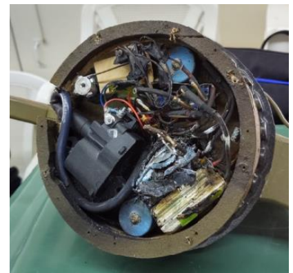
Damage from Lithium battery fire
